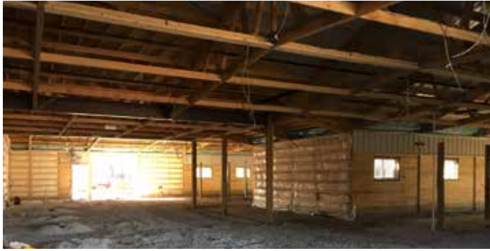
Interior construction progress
