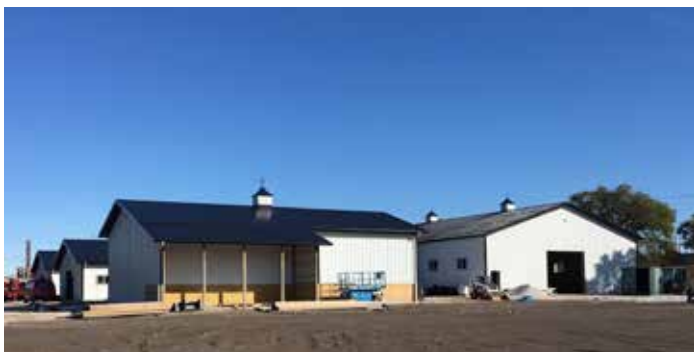
Exterior construction progress
