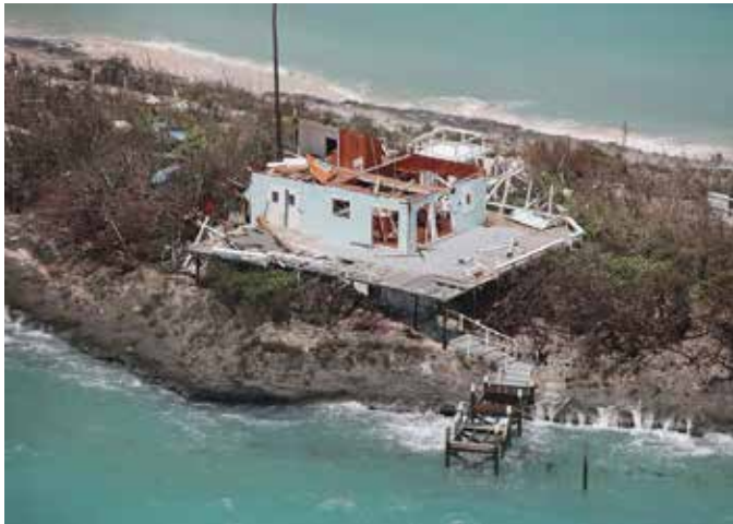
An aerial view of damage caused by Hurricane Dorian on Great Abaco Island in September.
