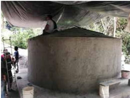
*The new suction tank that will hold water pumped up from the springs*
